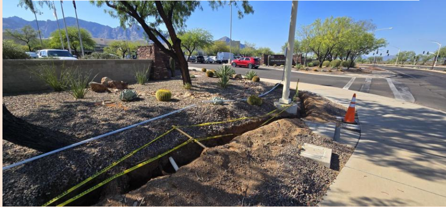
Assisting with irrigation installation
