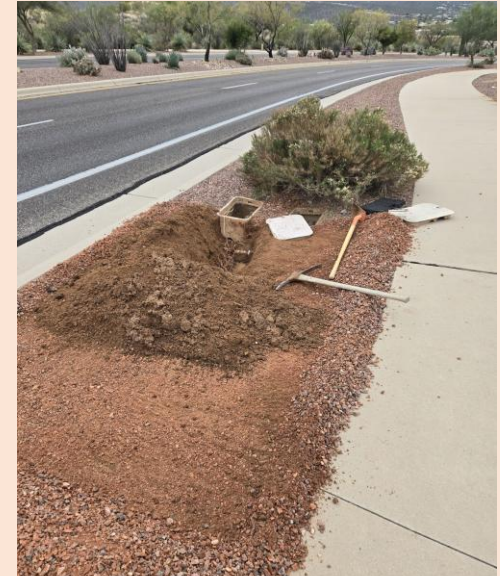
Irrigation line repair
